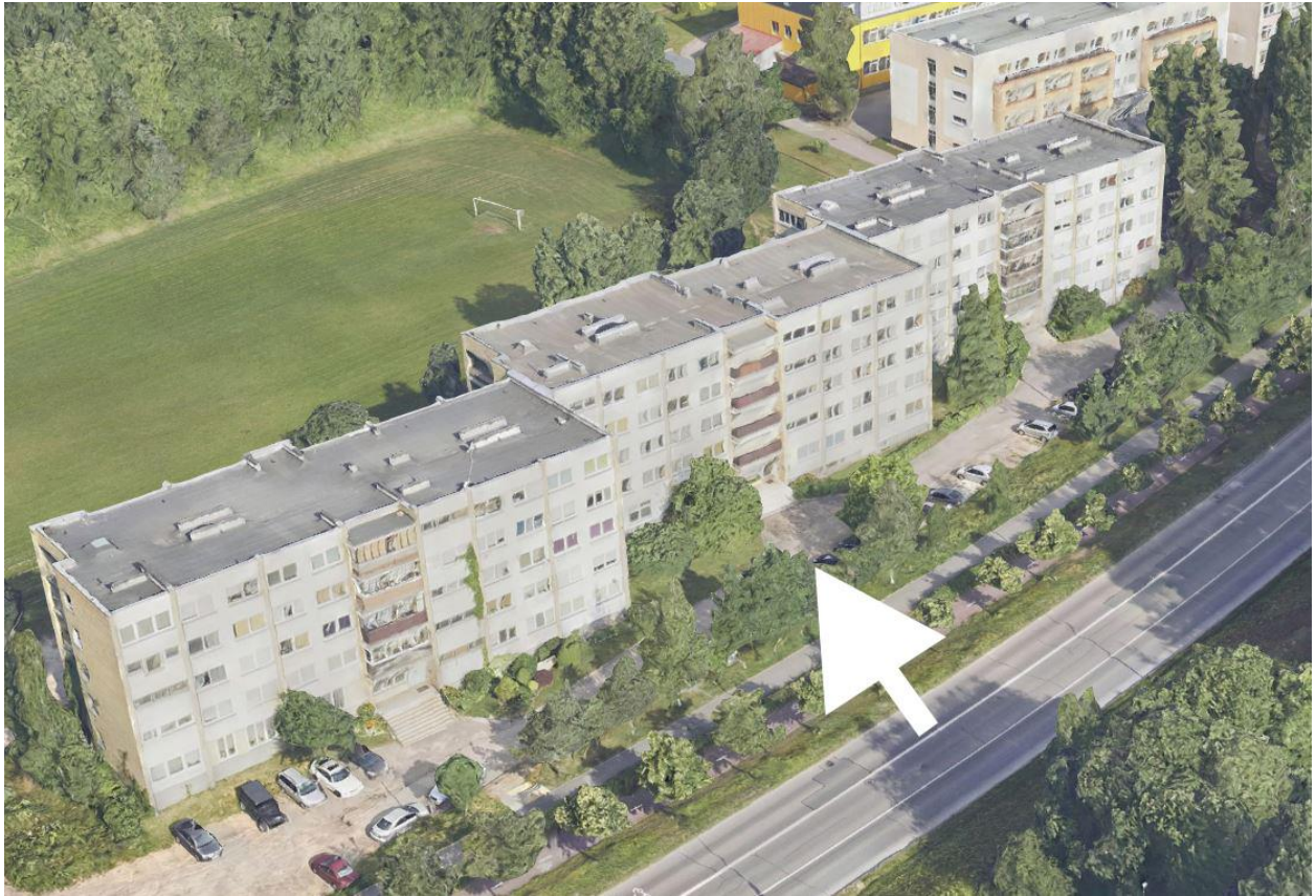
Picture 2 East façade and the main entrance.
