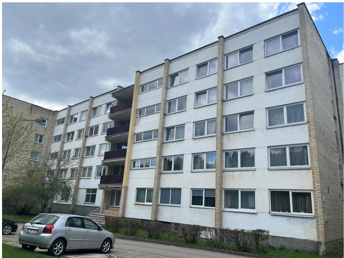
Picture 7 East façade.
