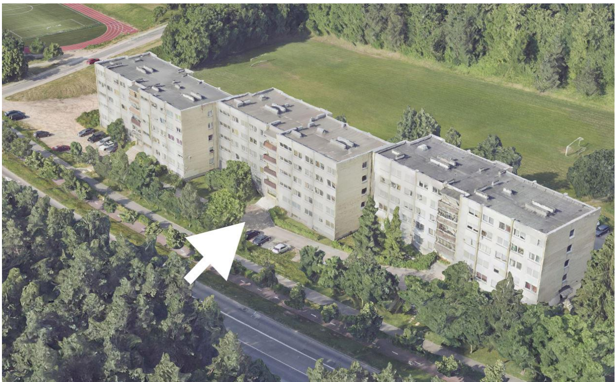
Picture 3 East façade.
