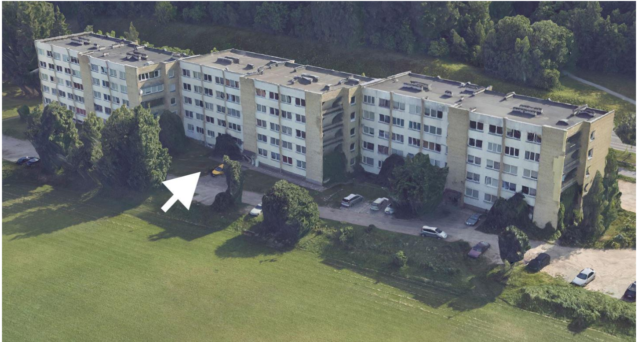
Picture 4 West façade.
