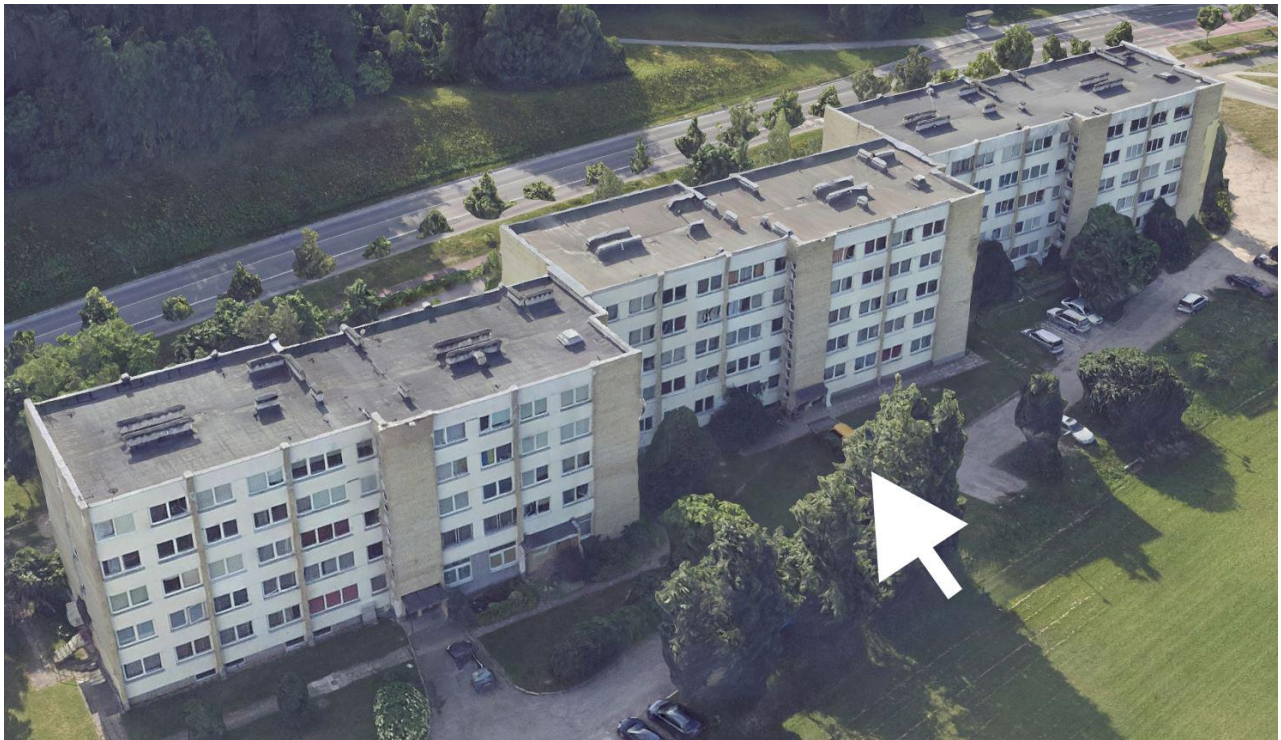
Picture 5 West façade.
